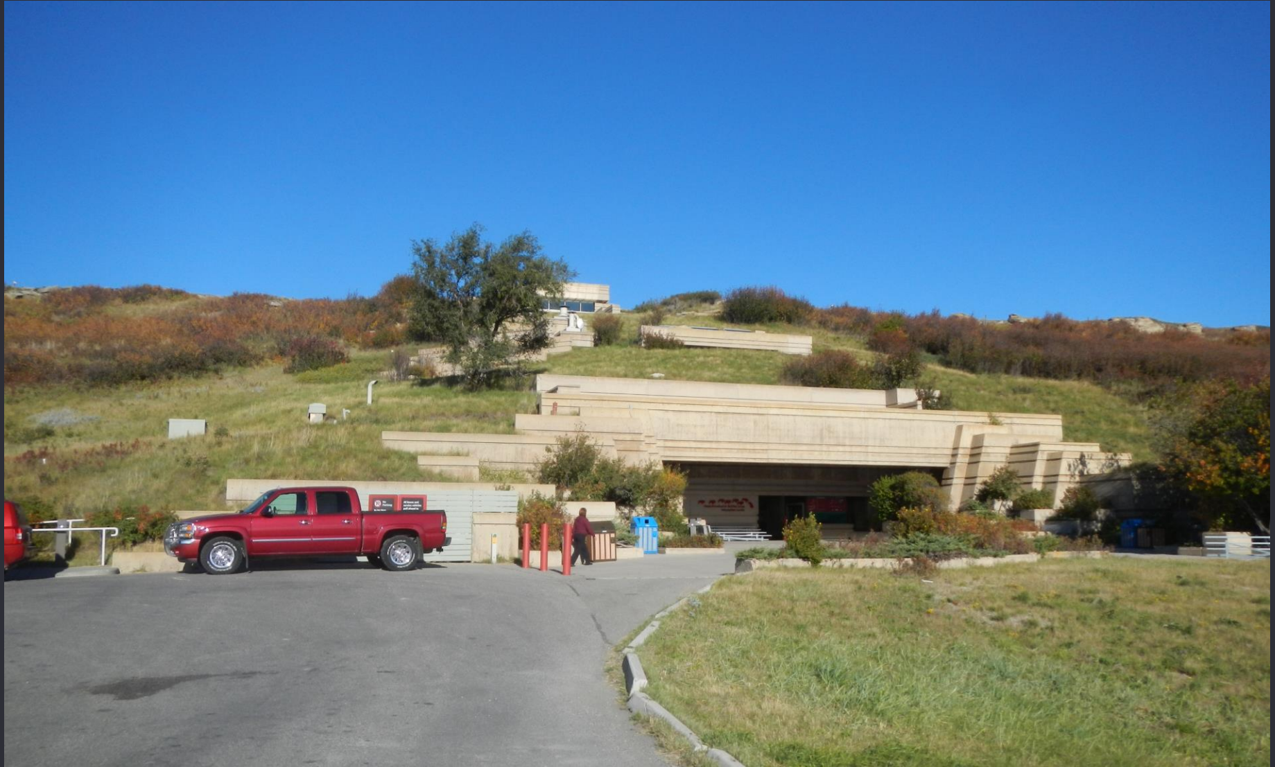
Entrance of the Interpretive Centre. View W.
